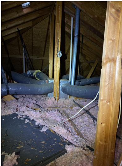
Overview of the AC/heating duct work
