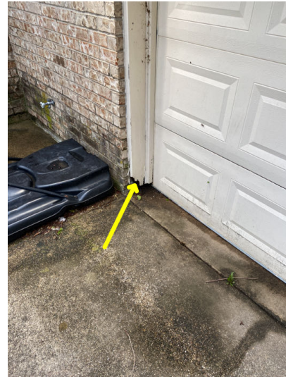
Both sides of the garage door have severe rot in the wood this needs to be replaced by a qualified contractor.
