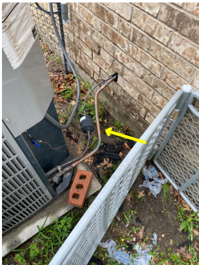
Damaged insulation on condensate lines should be repaired.
