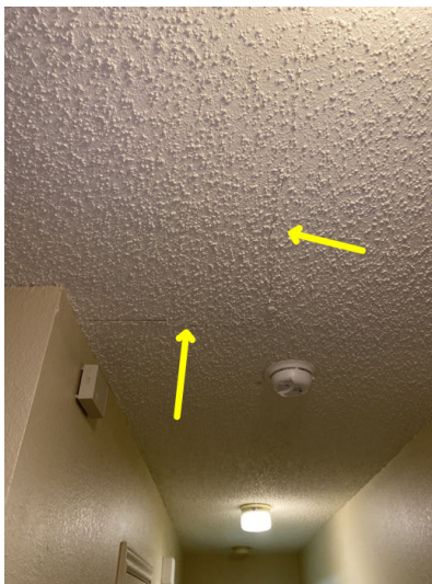
Cracking found in the ceiling in the front hallway leading to the bedrooms
