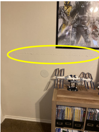
Horizontal crack found in the south central bedroom wall
