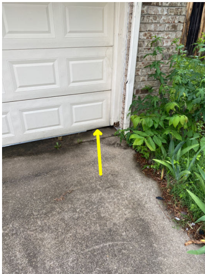
Garage door seal is torn and needs to be replaced.
