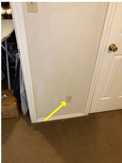
Loose outlet cover found in the master bedroom
