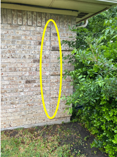
Vertical crack found in the brick veneer on the southwest corner of the house.
