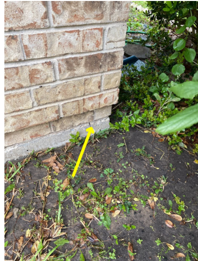
Minor cracking found on the southwest corner of the slab this is cosmetic in nature.
