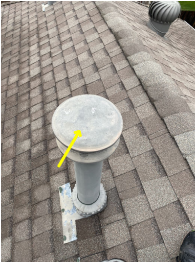
Minor dents found in the roof covering vent from previous hail damage.
