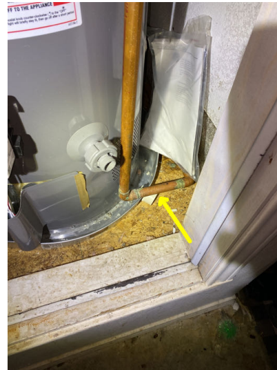
The drain pan drain pipe was not added during the installation of this unit it needs to be added by a qualified plumber
