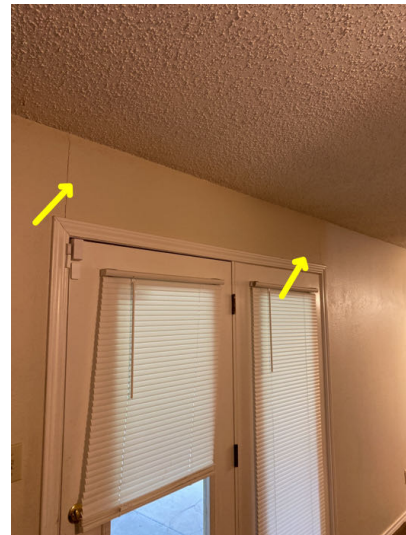
Wall cracks found above the back entry door
