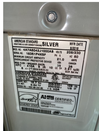
Outdoor AC unit specifications tag
