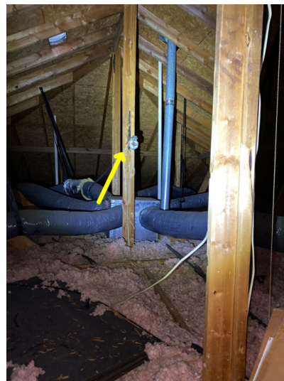
Open junction box needs to be closed off in the attic by a qualified electrician
