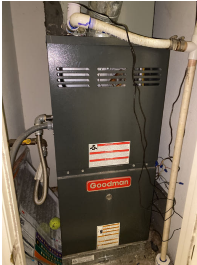
Overview of the indoor AC/heating unit
