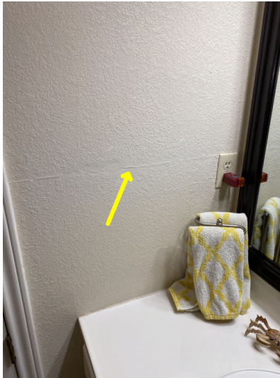
Minor wall crack found in the hallway bathroom
