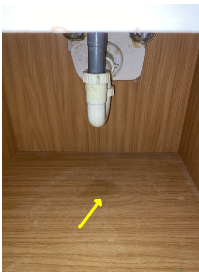
Minor leak found in the drain pipe underneath the hallway bathroom sink
