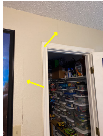
Vertical crack to the left and above the closet in the south central bedroom
