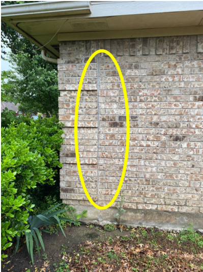
Minor settling crack seen on the south east corner of the exterior brick veneer
