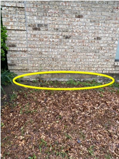
Additional backfill required on the south east corner of the slab to support the foundation.
