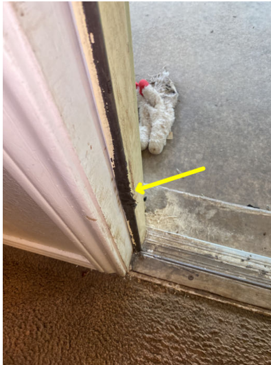
Torn weatherstripping found the back entry door
