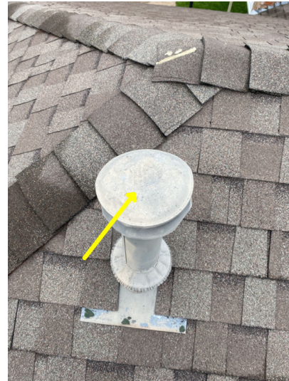
Secondary roof vent found with hail damage.
